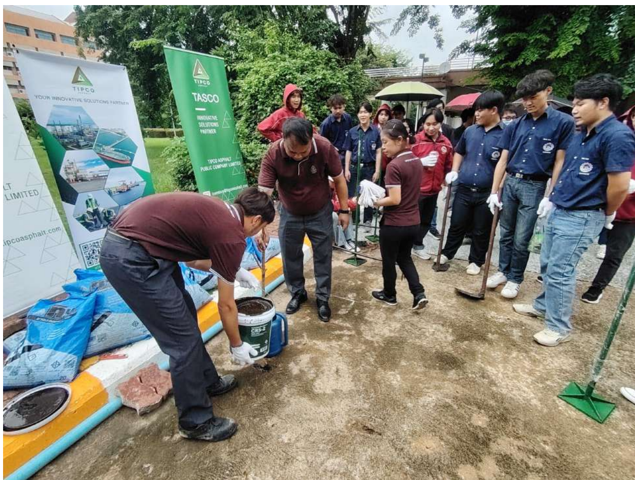
4.3 Improving the Entrance of the Faculty of Engineering, Naresuan University
