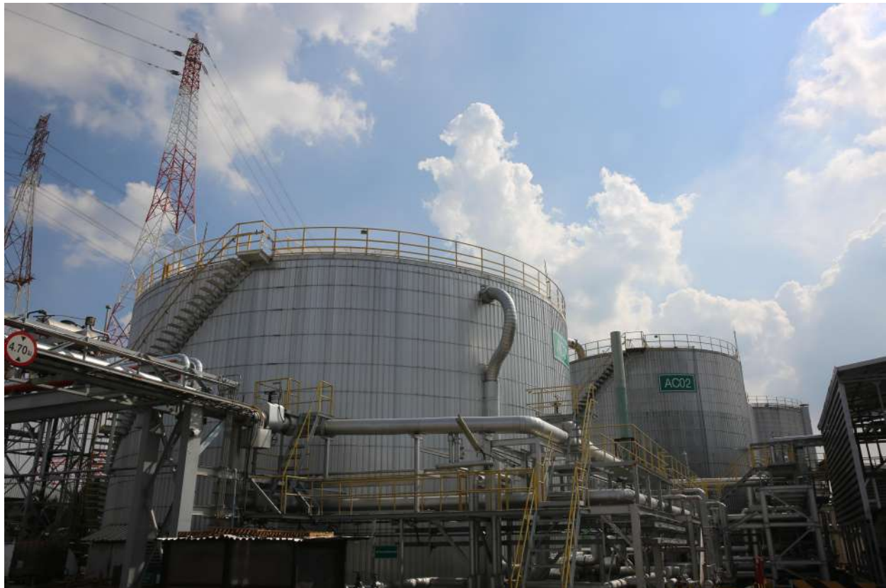
Thermal Insulation improving for preventing energy loss
