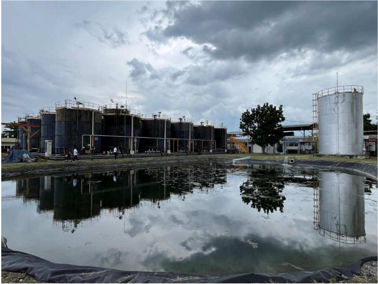
Water storage inside factory
