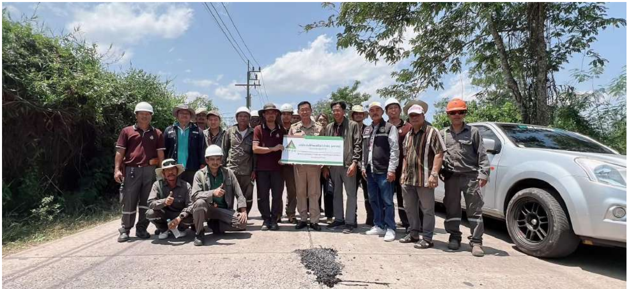
3. Project "Patching Potholes"
